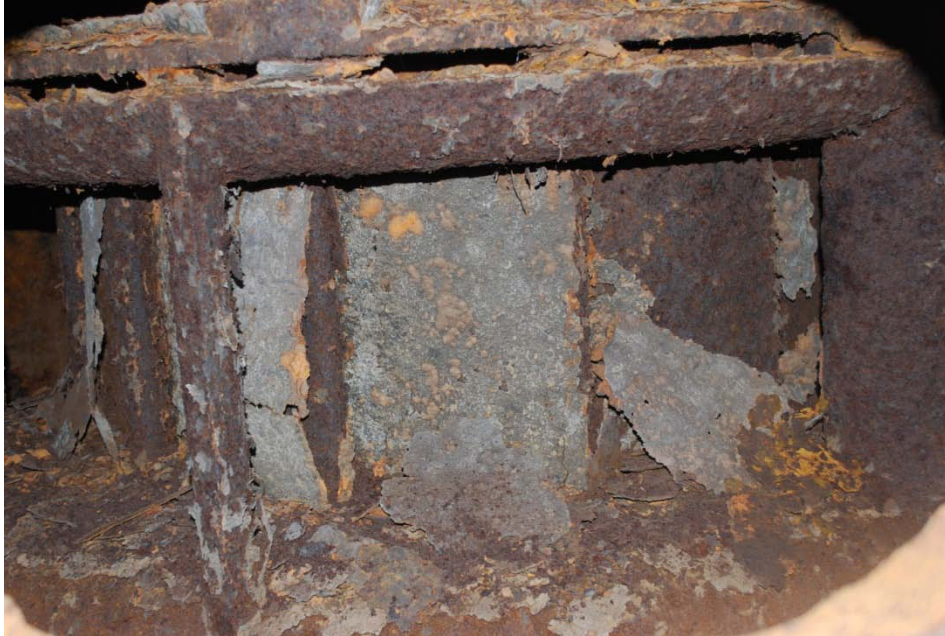
Figure 6. Headcover, Stay Vanes and Wicket Gate Assembly
