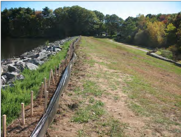
Photo 5. Turner Reservoir Dam. Left embankment from spillway.
