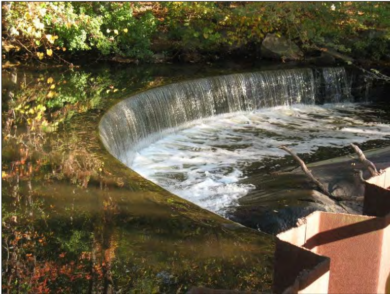
Photo 8. Hunt's Mill Dam. Spillway from right abutment.
