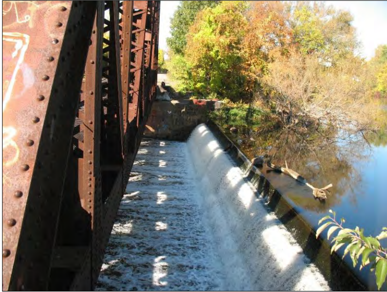
Photo 19. Omega Pond Dam. Spillway and right abutment.
