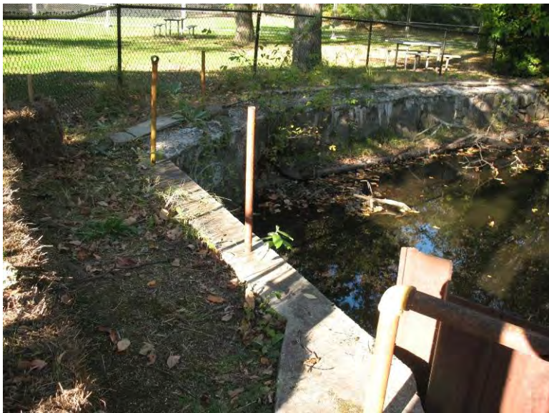
Photo 15. Hunt's Mill Dam. Retaining wall upstream of headrace entrance closure wall.
