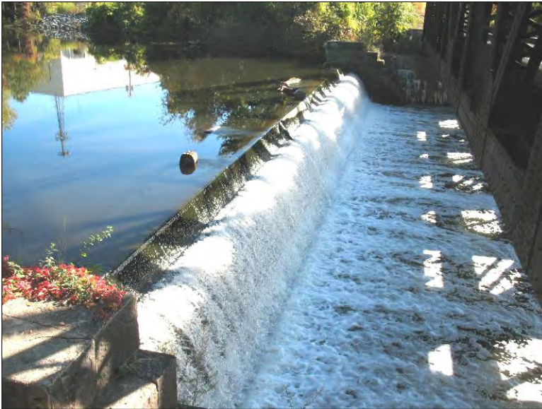
Photo 17. Omega Pond Dam. Spillway and left abutment.
